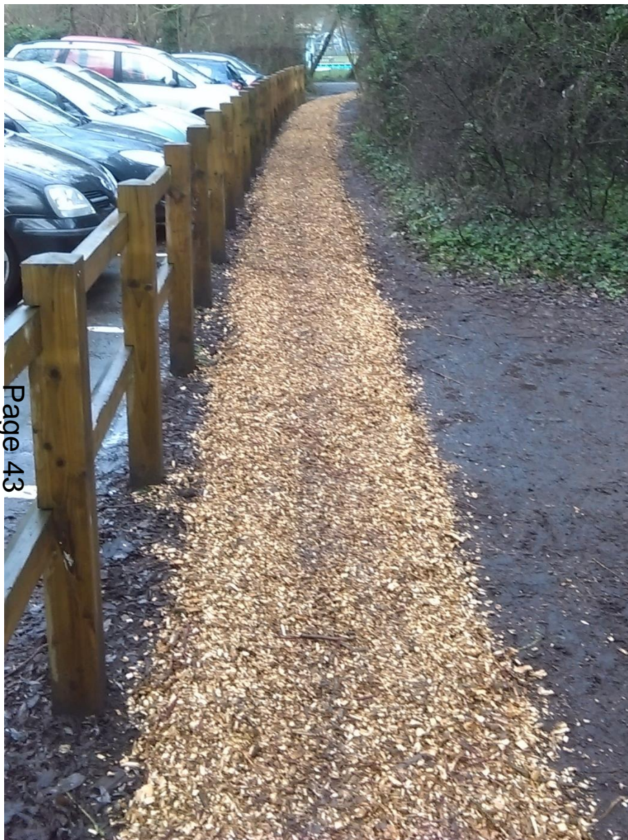
Photograph of works completed at Lammas Land car park
